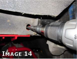
"self-align" the drill bit, forcing the bit to center itself in the hole.
